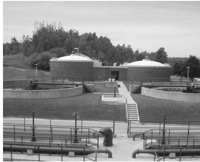
The Wastewater Treatment Plant will require several updates to meet State Regulations.
